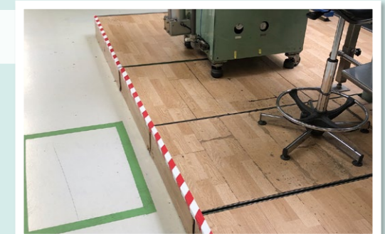
Labeling of hazard points on the floor
